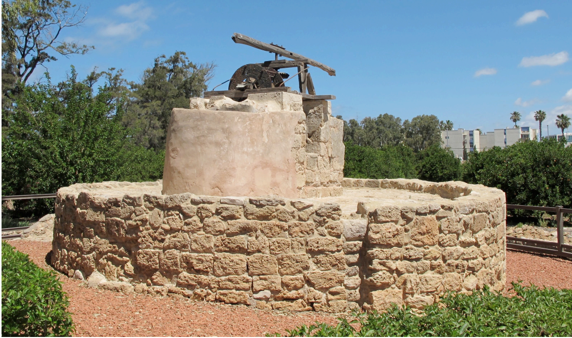
The water pump which pumped the water to the fountain and other parts of the garden. It was driven by a donkey.
